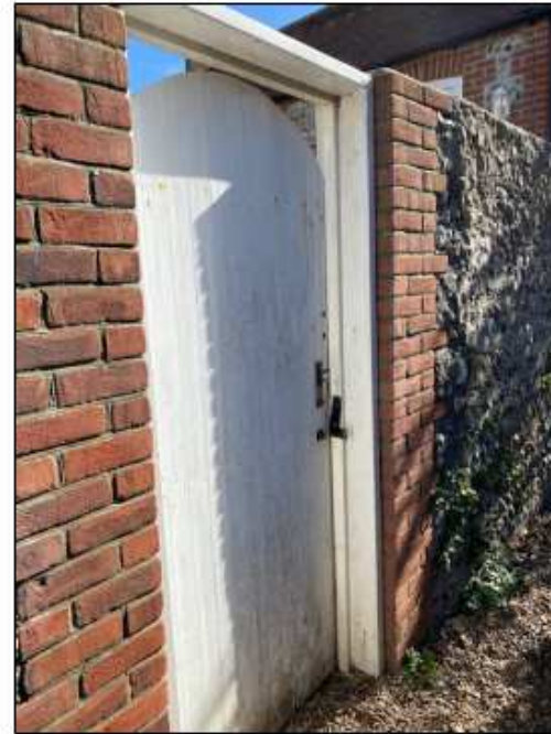
Existing entrance to annex from alley
